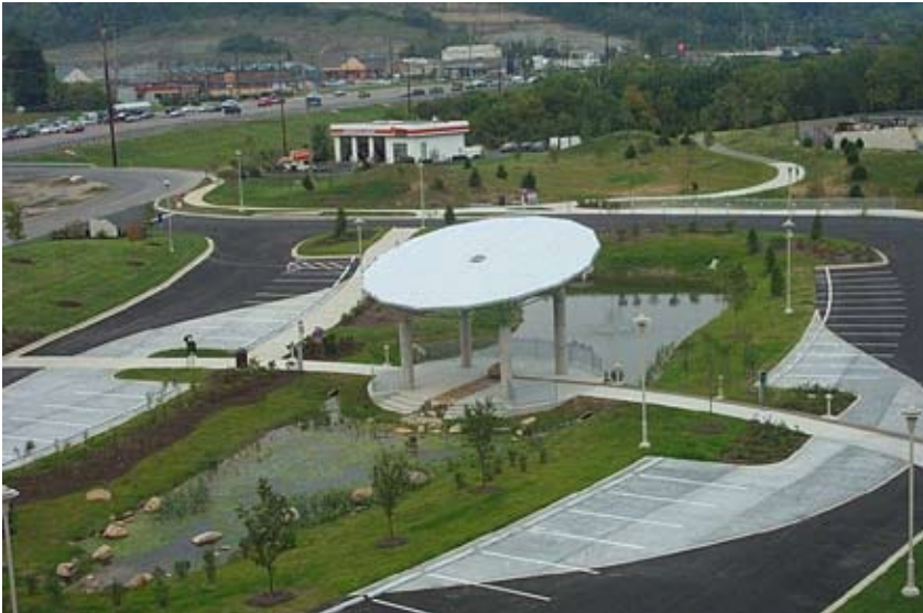
Sections of permeable asphalt and permeable concrete are demonstrated at Public Service Park.
